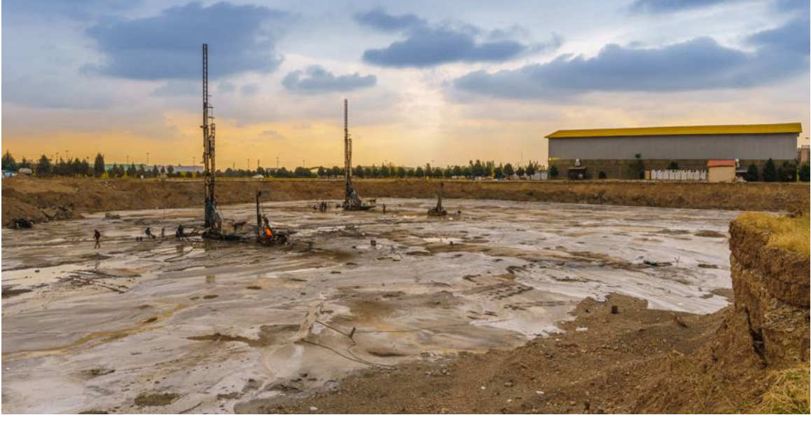
● Soil improvement project of Refah chain store by jet grout method
