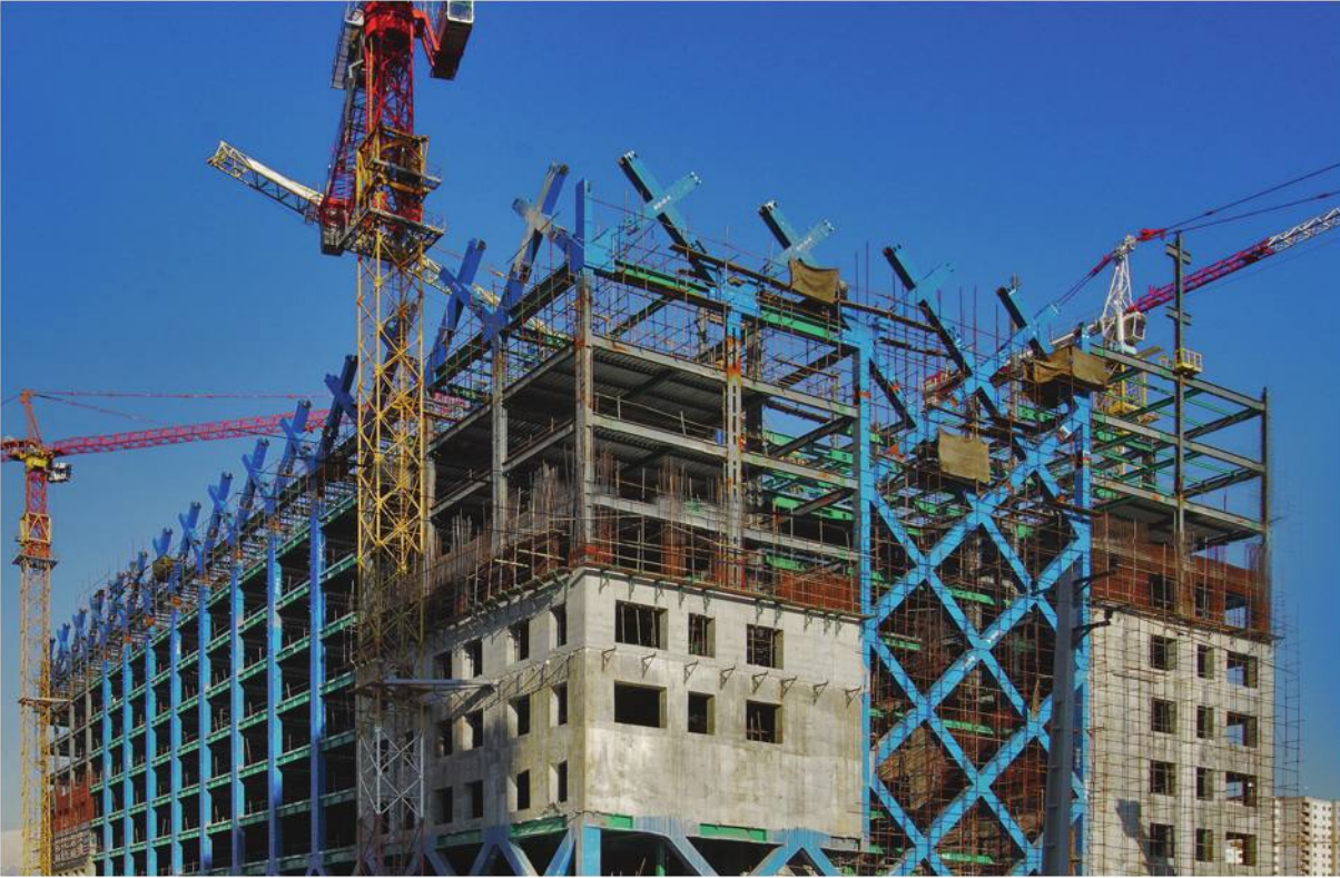
● The steel structure of Salamat-e Berekat hospital
