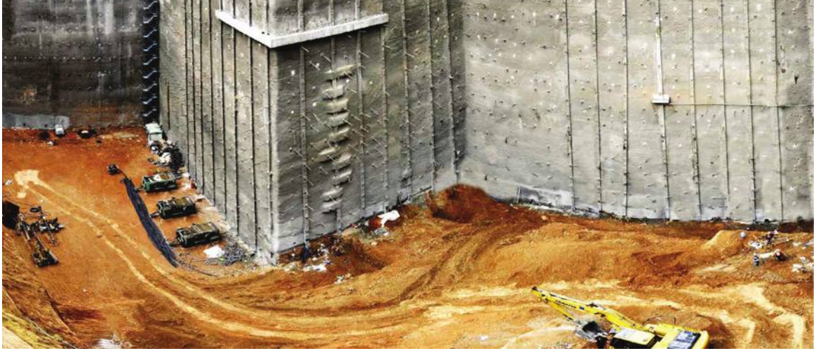
● Imam Reza multipurpose complex project
