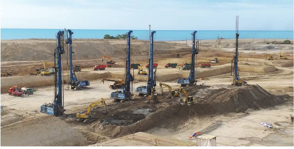
● Bushehr soil stabilization project
