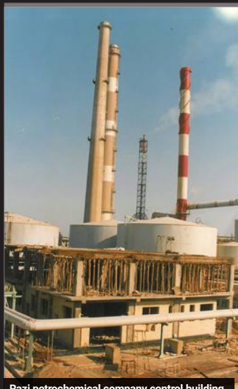
Razi petrochemical company control building
