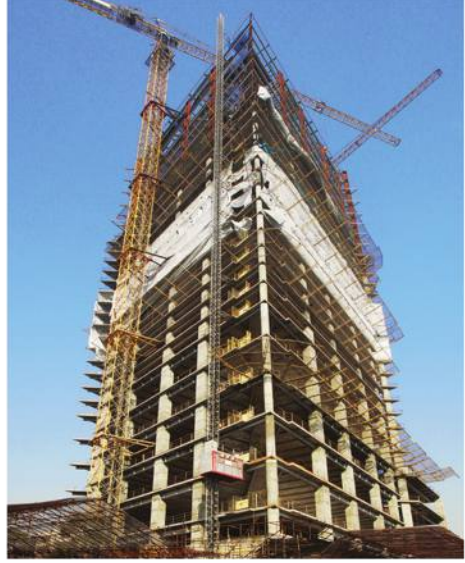
● The steel structure of Metal Hotel
