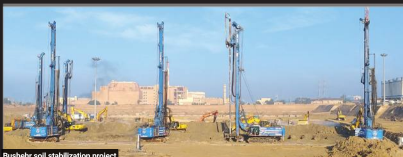
Bushehr soil stabilization project
