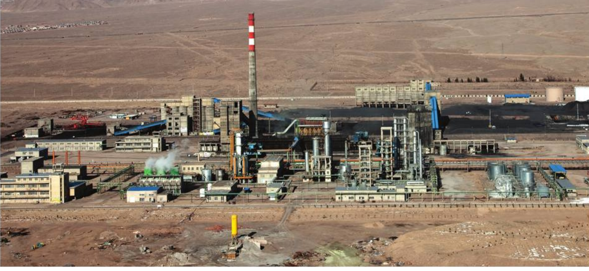
● Zarand coke production and Tar refining factories
