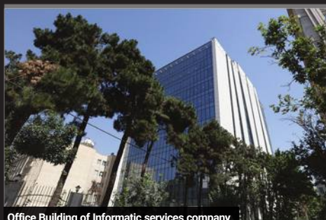
Office Building of Informatic services company
